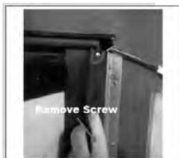
Figure 8 Removing the bulb seal screw
